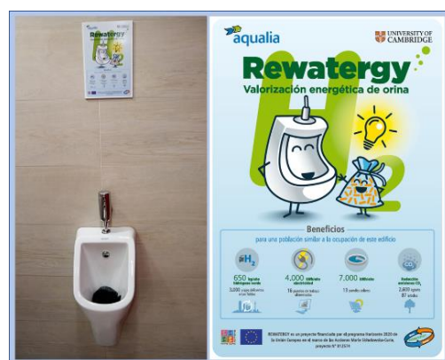
Photo at the left, urinal with activated carbon installed in Aqualia's office in Madrid. Photo at the right, detail of the picture deployed next to the toilets with the REWATERGY solution.
